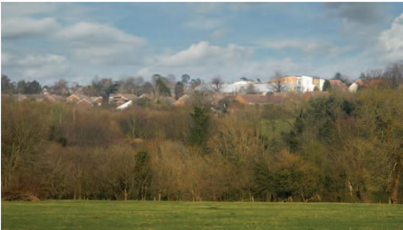
Where town meets country - the western boundary of the North Loose area where it meets the Loose Valley Conservation Area
