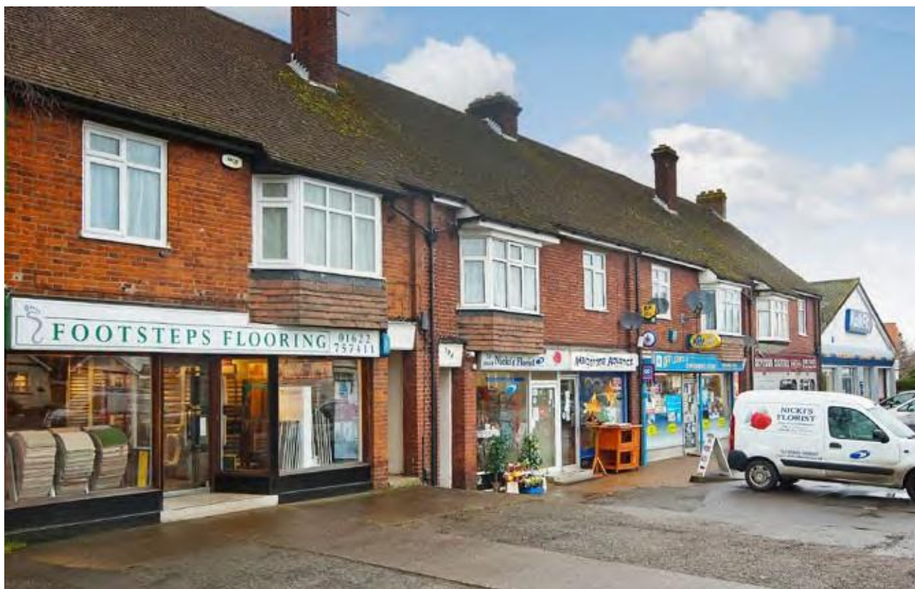
Scope to improve public realm in front of parade of shops
